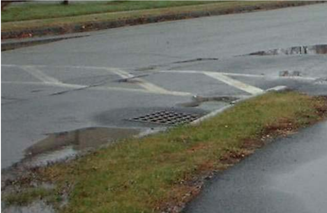
Figure 6-Ralph Lehman Road Existing Drainage
